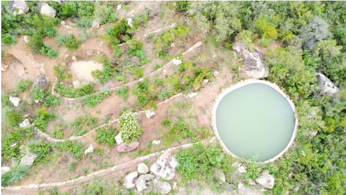
AAF in Sipe Sipe (the farm): agroforestry, contour lines, 1 water reservoir and 2 water infiltration lakes.
